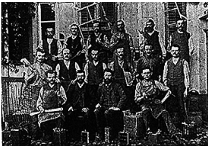
Group of workers of the Rosport factory with the different models of the Tudor battery at their feet.
